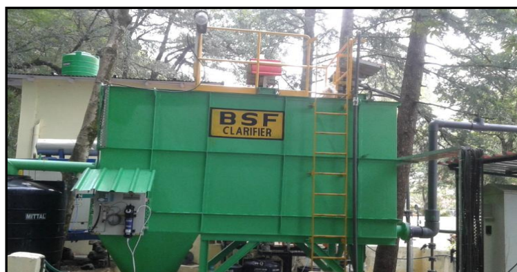
Figure 2. Actual experimental set up (1 Mld pilot-plant) at Nainital, India
