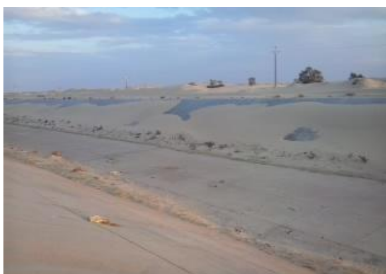
Figure 6. Sand accumulation in EL-Sheikh Gaber Canal at km 63.000.
