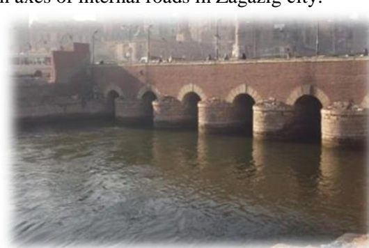
Figure 2. Photo of the ninth barrage
