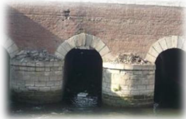
Figure 6. Falling of some of the building bricks/stones as well as disintegration of taban fence
