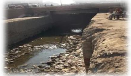
Figure 8. Not pitching the lock inlet and falling rubble debris into the waterway
