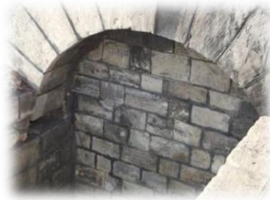
Figure 13. Block opening No. (1) entirely from the front by wall building
