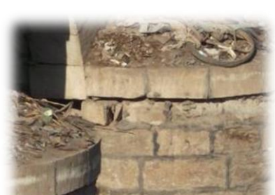
Figure 8. Not pitching the lock inlet and falling rubble debris into the waterway
