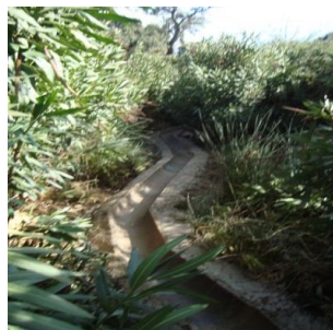
Figure N° 5 : Realization of irrigation canals
