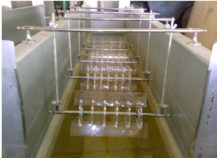
Photo 1: Installation of self-RBC discs on the channel
