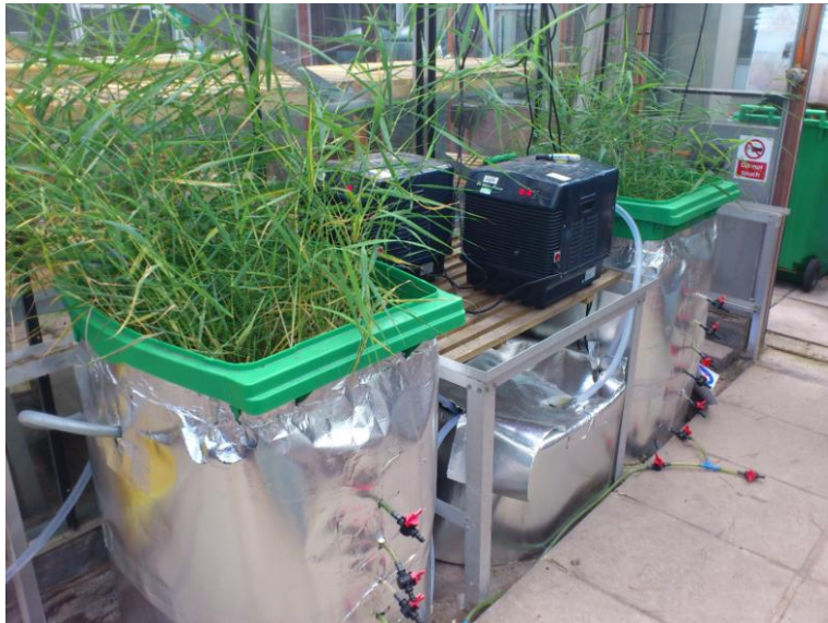
Figure 3: Photograph of combined constructed wetland and SWHP (I) and stand-alone constructed wetland system (II) taken October 2011, after four months into operation.
