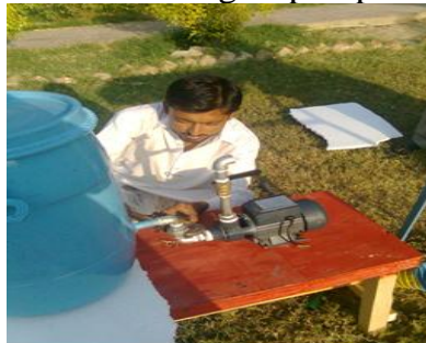
Figure 7. Fitting of pump
