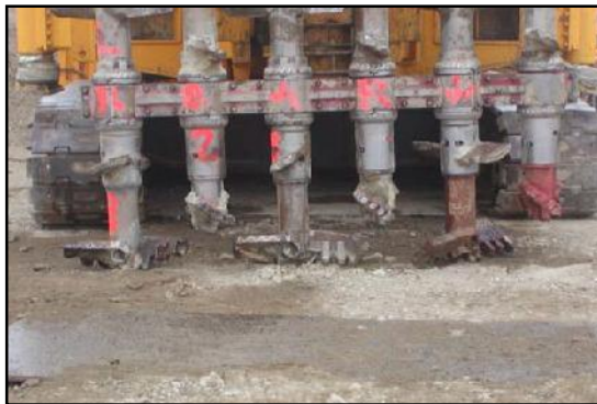
c) Soil mixing machine
