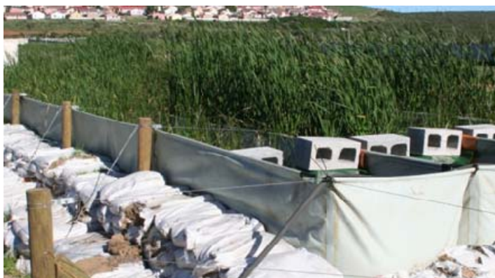
Figure 1 (A) The high rate algal ponding system with primary facultative pond, and hydroponic system in the background and (B) the constructed wetland.
