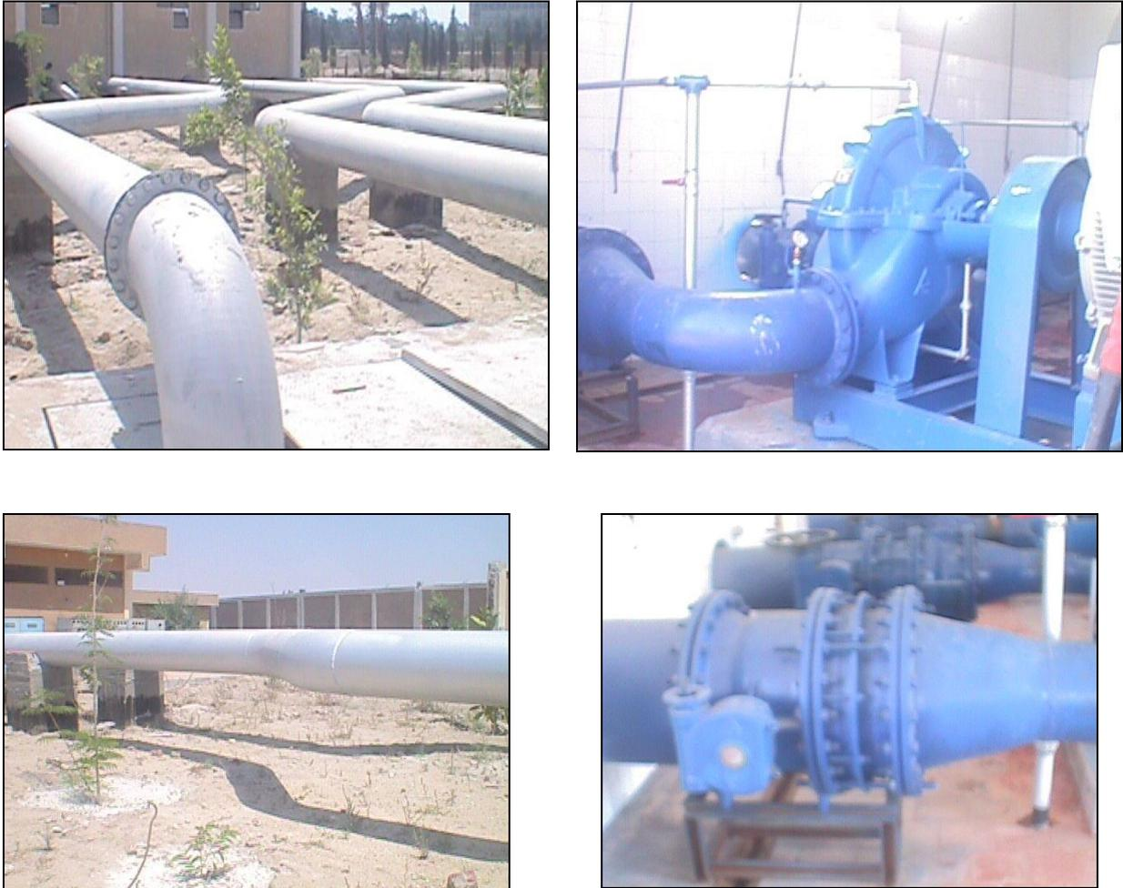
**Figure (5) Suction pipe, pipe reducer and elbow at pump suction**
