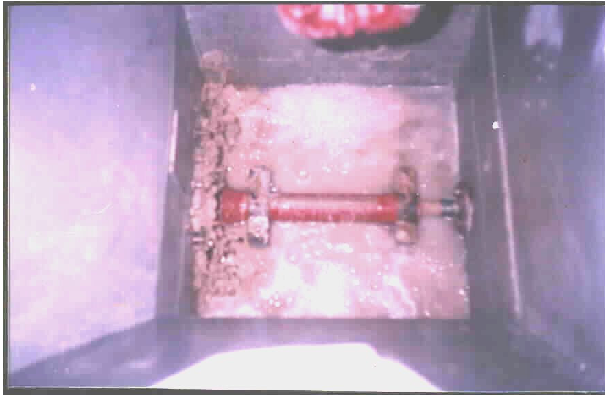
Fig. (3): Photograph of top view of the aqua jet pump scrubber where partition which separates between the two chambers [I] & [II]
